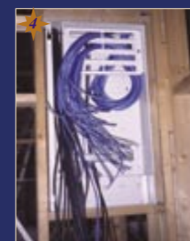
Cabinet is fixed in wall.
