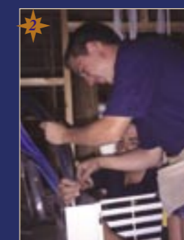
Cables are passed through entries on cabinet, ready to be mounted into wall.
