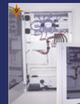
Second fixing to StarServe cabinet complete.
