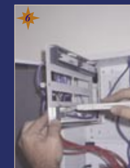
Terminating Cat 5 using Krone tool.
