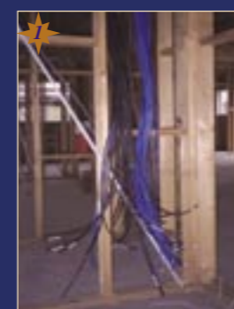
Layout of cabling completed and running back to StarServe hub in preparation for installation of cabinet.
